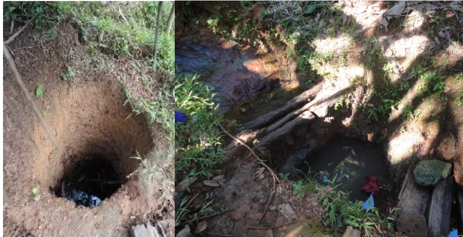
Figure 9: (a) Hand Dug Drinking Well (b) Partitioned Drinking (upper) and Washing (lower) Unimproved Well Sources in La Ensenada
