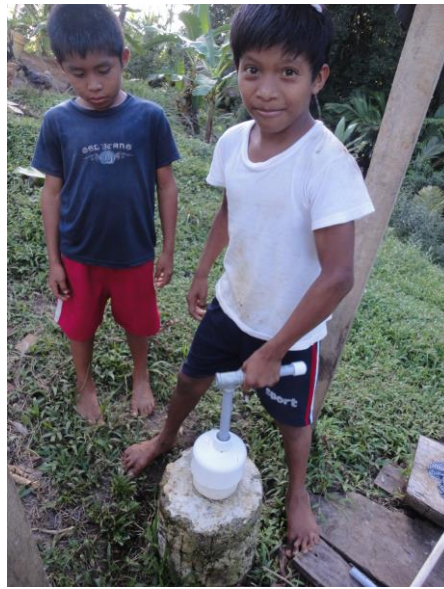
Figure D.4: Broken Handle of EMAS Pump at Attachment between Galvanized Iron “T” and PVC Half Inch Pipe La Ensenada
