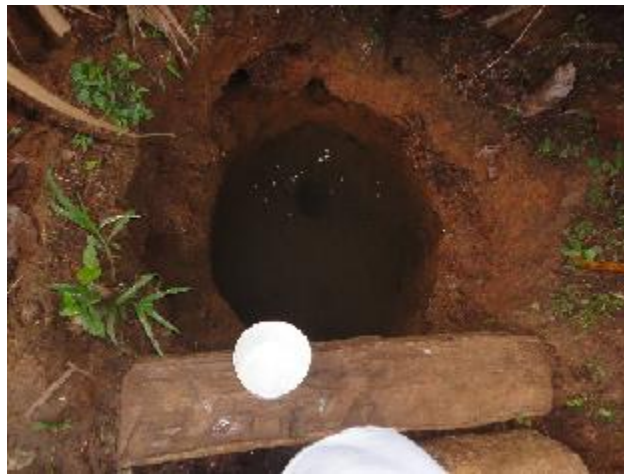
Figure D.2: Unimproved Drinking Water Source and Water Scoop Top View (which demonstrates soil and depth characteristics)
