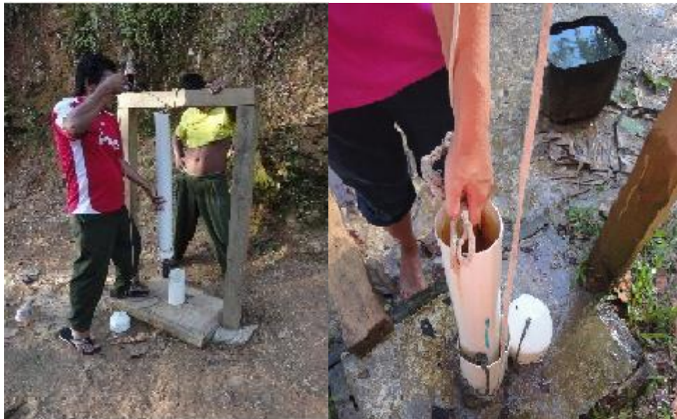
Figure 10: (a) Bailer Demonstrated in La Ensenada (b) Bailer System Top View
